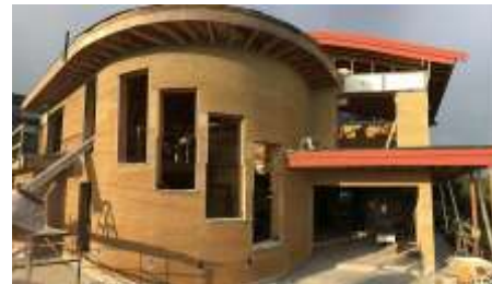
(Figure 13) Hemp-crete installation at the Highland Hemp House Project in Bellingham
