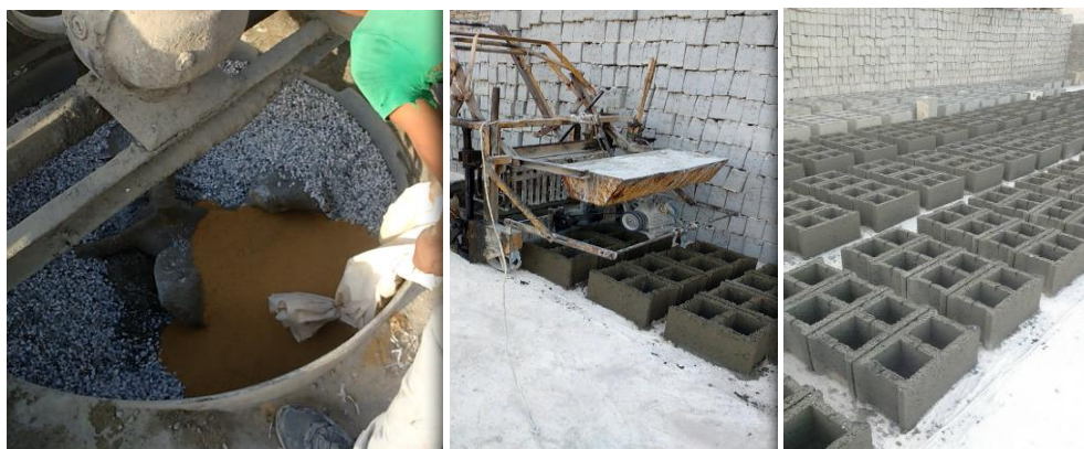
Fig (2) show the production process of hollow concrete blocks.
