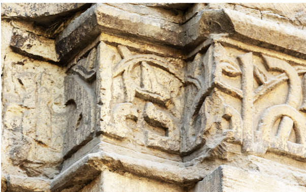
(Fig. 9) Cairo, Mosque of al-Aqmar (1125), details of the upper (top) and lower (bottom) foundation inscriptions on the façade.
