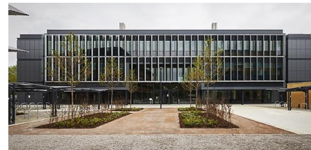
Figure 13: Applying thermochromic glazing in the Civil engineering facades, Cambridge University, United Kingdom, to maintain thermal comfort [18]
