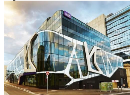
Figure 14: Thermochromic glazing facades of NDIA headquarter, Geelong in Australia [20]
