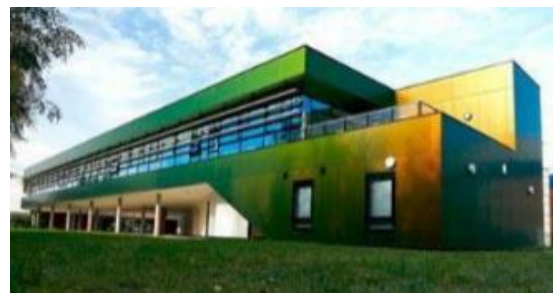
Figure 25: The chameleon decorative panels at Think Tank Innovation Center facades, Lincoln University, United Kingdom [34]
