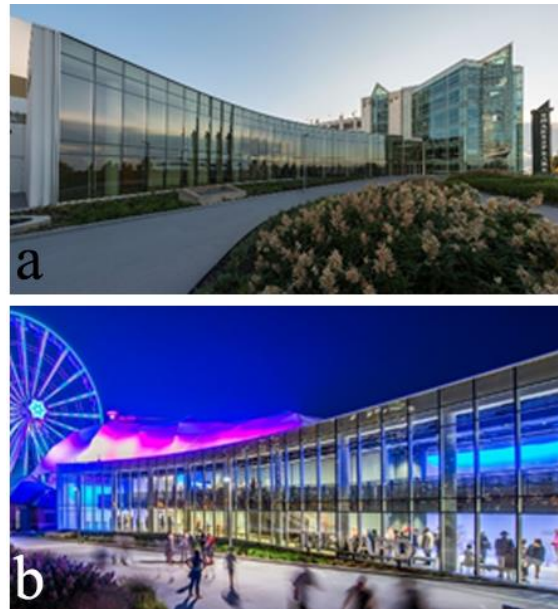
Figure 18: Electrochromic glazing is used in the south façade of the Yard, Chicago Shakespeare in USA (a) the facade is opaque at daytime to control heat gain and (b) the glazing façade is transparent at night [26]
