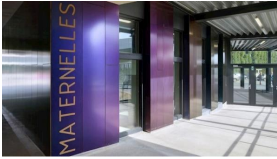
Figure 26: The chameleon decorative panels at Les Trèfles primary school in Anderlecht, Belgium, Europe [35]
