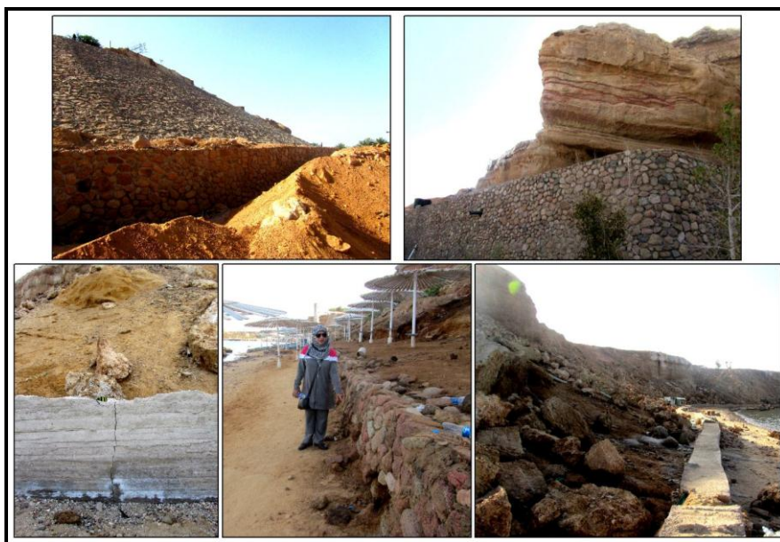
Figure 18. Some of the protection methods from the hazard of rock falling from the marine scarp of Um Sid Plateau.
