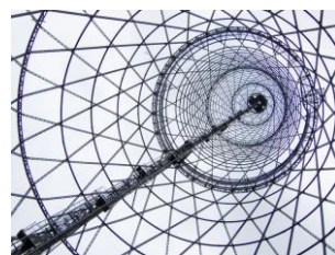
Fig. 5. Diagrid structure of Shukhov Vladimir metal tower [4].
