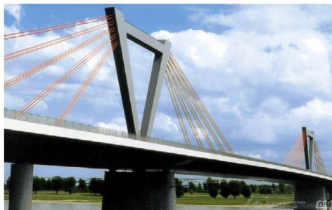
(b) The Ilverich Bridge in Germany
