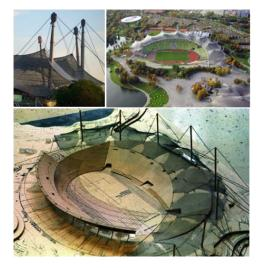
Fig. 11: Munich Olympic stadium, Frie Otto, 1972. The Stadium makes extensive use of tensile roofing construction [25, 26]
