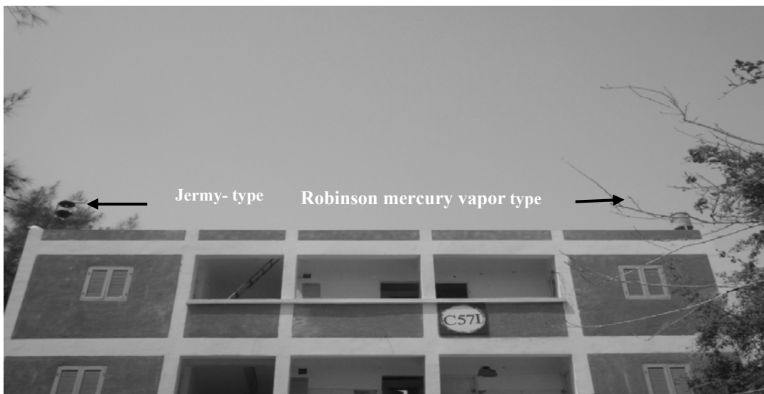
Robinson mercury vapor type and Jermey type light traps above the roof of Irrigation station (Building No.C571).
