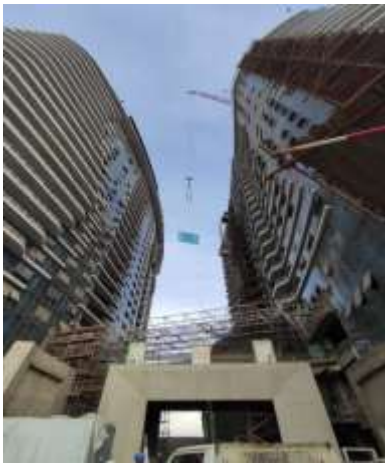
Figure21 : 1 crane ready to transport materials (before)
