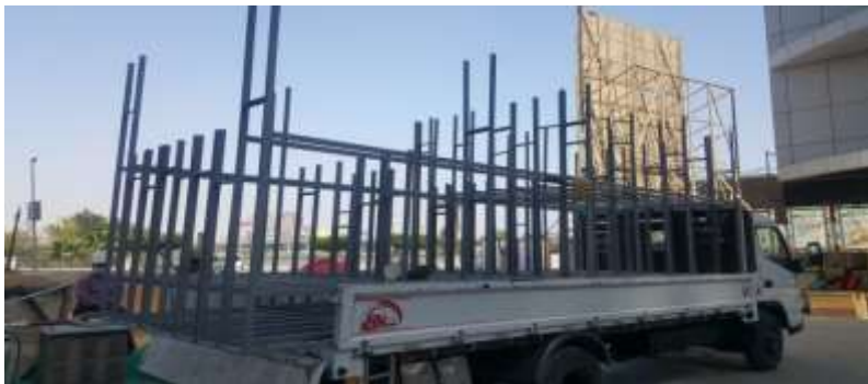
Figure 15 (up) : arriving materials to the site
