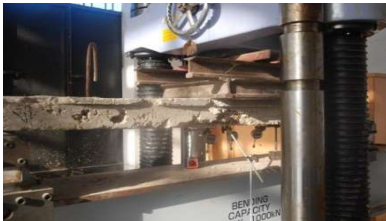
Figure 7. Corrosion pattern in RC beam B2.
