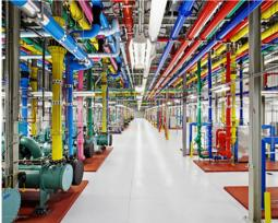
Figure 11, Using color for pipeline classification Kamitopen: 2020
