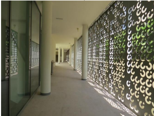
Figure 20- The Southern Façade shows the Architectural solution to decrease the building Heat Gain. (Source: Bit-Design Architecture Office, 2020)
