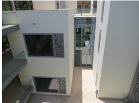
Figure 19- Building form creates shaded patio to the Class Rooms. (Source: Bit-Design Architecture Office, 2020)
