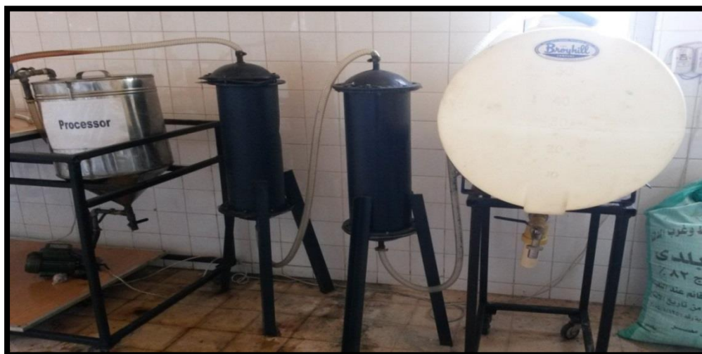
Fig. 3. Dry washing filters
