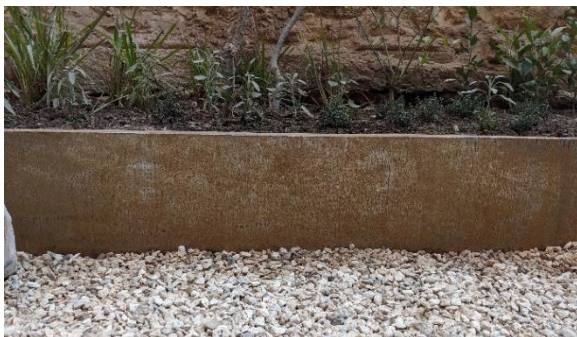
Figure 19: Rusting finishes of the steel [Source: Researchers]
