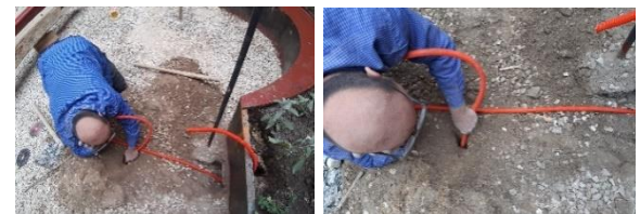
Figure 30: The electrician passes the wire through the plant's soil to the underground tunnel during the implementation process. [Source: Researchers]
