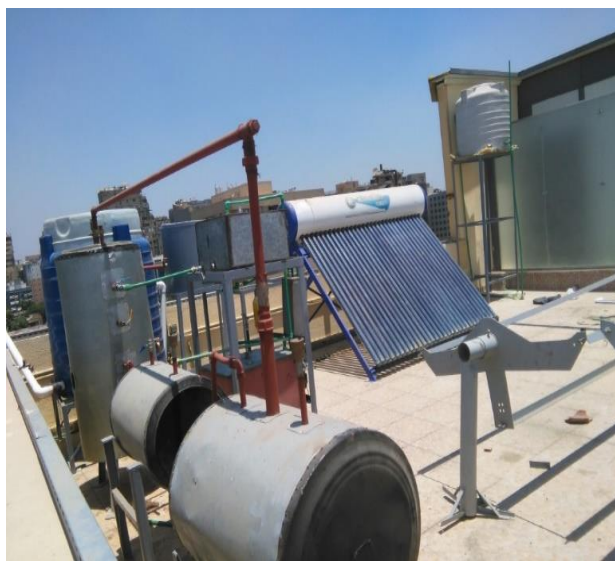
Fig. 2 Photographic view of a solar water desalination system using evacuated tube collector [31]
