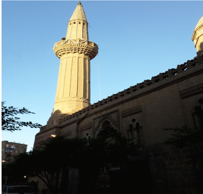
Facade of Šeiḥ Sāleh Ābū Hādīd Mosque photographed by the researcher
