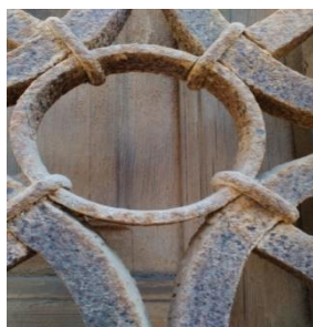
Fig. 3: Window grille components were joined by using iron collars, rivets, and connectors.
