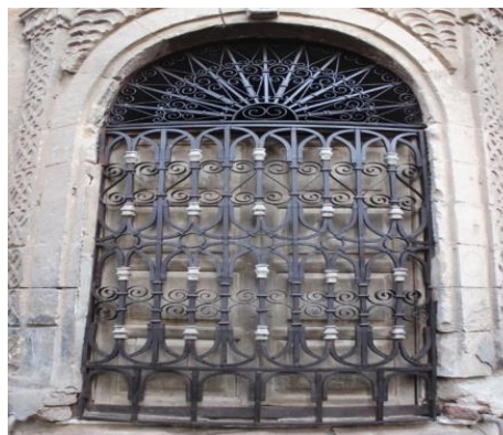
Fig. 10: The iron window grille after conservation treatments
