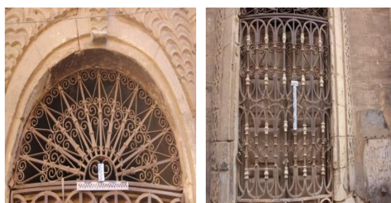
Fig. 1: Represents the iron window grille of sabil Ramadan and documentation by drawing of the window grille shows the twenty lead connections are still existed.
