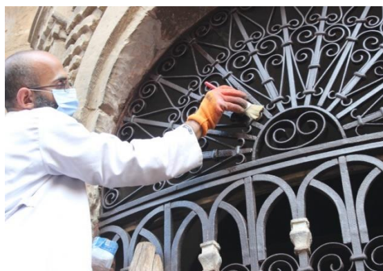
Fig. 10: The iron window grille after conservation treatments
