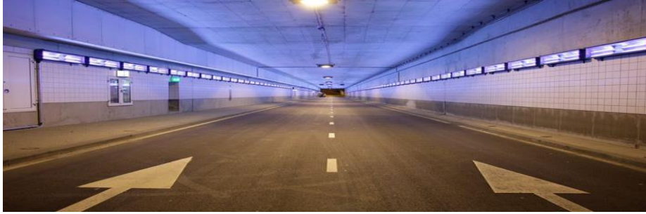
Figure 1٣: The Hague performs an innovative environmental experiment in the Konings tunnel, May 22, 2013. (30)
