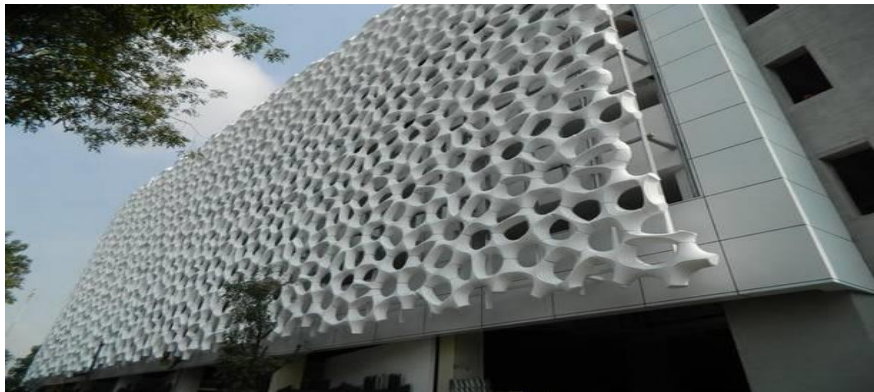
Figure ٧: The Manuel Gea Gonzales Hospital in Mexico City installed a hive-like facade painted with KNOxOUT to purify the air that enters the building. | Photo Credit: Pacific Paint (Boysen) Philippines. (24)
