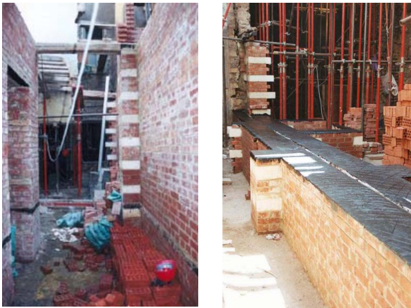
Fig. 3- The wide sidewalls between houses Source: the Author, (2003-2004)
