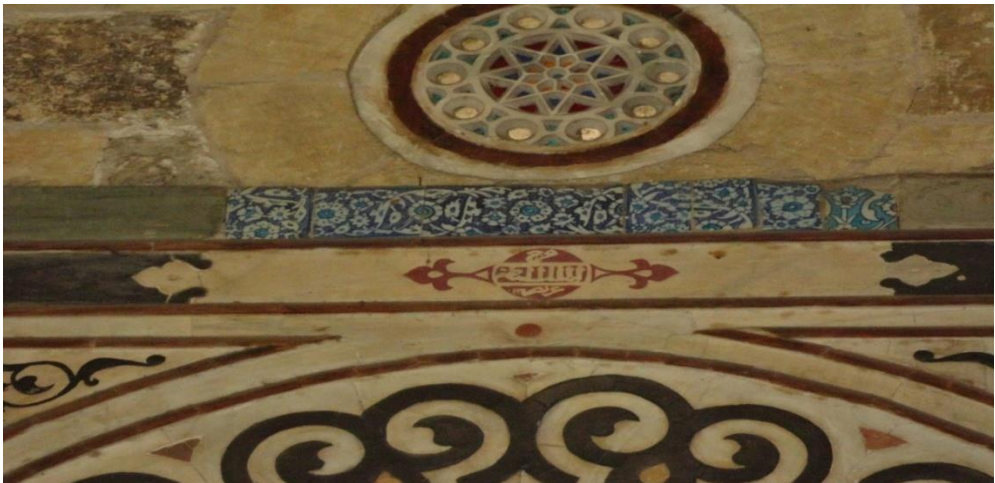
PL (5) : Cairo, Qasabet Radwan Street, the era of the Mameluke Circassian, Al-Sultan Al-Nasir Faraj ibn Barquq mosque, Three heraldries of Sultan Faraj ibn Barquq, in a joggled marble bar in black and white inscriptions on the mihrab's squinch in the south-eastern wall of Bayt al-Salah, on a red colored background, 811 AH/ 1408 AD
