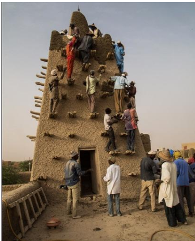
Figure (10) Shows climbing on wood pieces during restoration - Djinguereber mosque in Timbuktu, Mali. (After, https://www.flickr.com/photos/minusma/32239632874 , 4/03/2020)
