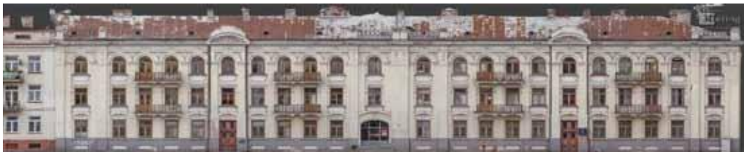
Figure 56. Historic Elevation in Plock in Plock, Poland (“Historic Elevation in Plock,” 2018).
