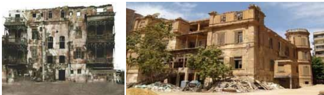
Figure 1. Demolition and neglect of architecture heritage in El Max, Alexandria and Villa Ambron, house to the great British author Lawrence Durrell (“Villa
