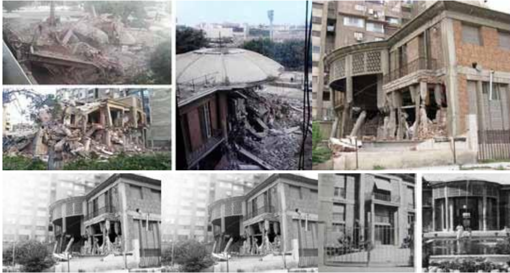
Figure 3. villa Aghion design after the collapse in Alexandria.
