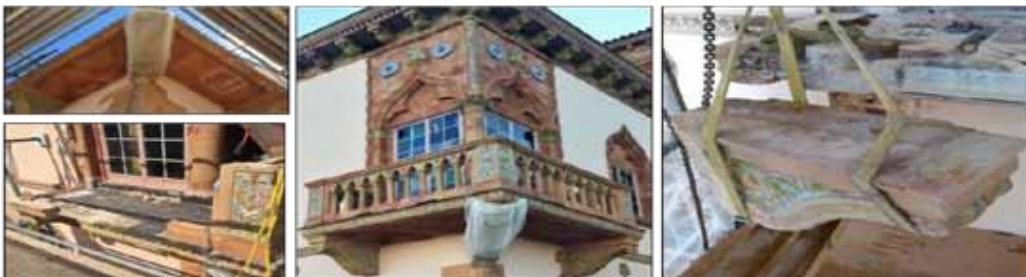
Figure 8. ORNAMENTAL TERRA COTTA RESTORATION - RINGLING MUSEUM
