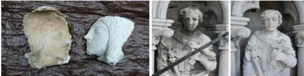
Figure 6. Modeling Replacement for Sculpture Losses, Sculpture Conservation, Face Replica. The project showed a hard shell formed on the outside of many sculptures, while the basic stone materials have been eroded leaving only loose grains. The cracks formed on the surfaces to expose the damaged interior to the water and caused the full elements to fall (Figure 7). Materials / Limestone, Mortar.
