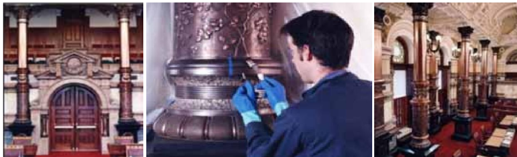
Figure 12. Bronze Columns at the Kansas State Capitol Senate Chamber, Metal Architectural Elements at the Kansas State Capitol Senate Chamber, Bronze Conservation Treatment. The Senate Chamber was a unique artistic work ornamented in 1885. The round windows, which feature faceted stained glass, were imported from France. The walls were decorated with various exotic materials from all over the world. The research team reviewed historical documents, besides, conducted on-site tests to determine the original appearance of metals and their degradation and cause nature (Figure 11). The 28 columns were ornamented with ornate panel, decorative ornaments and wall grids so that all surfaces could be accessed. Old protective coatings and corrosion products have been removed from copper, silver and the missing parts have been removed and re-installed. Large areas of loss of paint and new castings were replaced on site using brushing technique (Figure 12) (“SENATE CHAMBER METALS CONSERVATION - KANSAS STATE CAPITOL project,” 1999). Materials / Electroplated Cast Iron, Stamped Copper, Cast Bronze, Nickel/Silver. Services Provided / Surveys-Condition Assessment, Research-Documentation,
