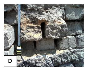
Fig. 6. A. Falling of the covering stone layer from the pyramid, B. Al-Ibrahemeya canal which affect the pyramid and the archaeological site. The arrow indicatesthe location of the adobe pyramid, C and D. show the collapse and erosion of adobe blocks due to windstorms and other environmental factors.
