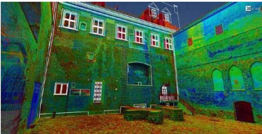
Figure 53. The building was scanned at the highest resolution settings for all external interfaces. Then, it was covered by the CAD with Orthoimages to show the full potential of laser scanning (“3Delling - 3D Laser scanning,” 2018).
