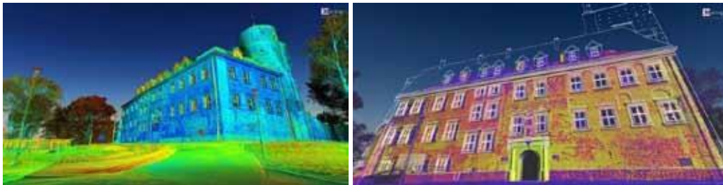
Figure 55. Survey work and a three-dimensional visualization of the site were produced.
