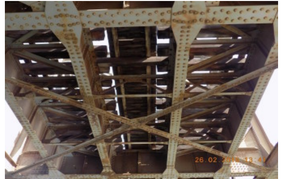
Figure 14. Addition of Stringer Bracing, Banha Bridge
