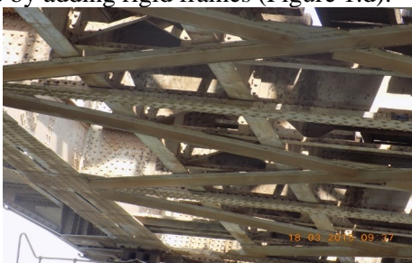
Figure 13. Replacement of Lower Bracing Members, Mansoura Bridge
