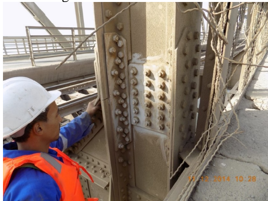
Figure 15. Replacement of Vertical Truss member after Train Derailment Accident, Marazek Bridge
