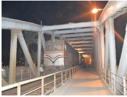
Figure 11. Static Load Test, Zefta Bridge
