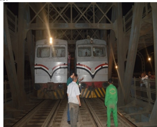
Figure 10. Static Load Test, Imbaba Bridge
