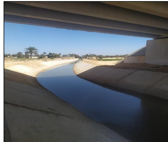
Photo (1): Lining works in the canal
