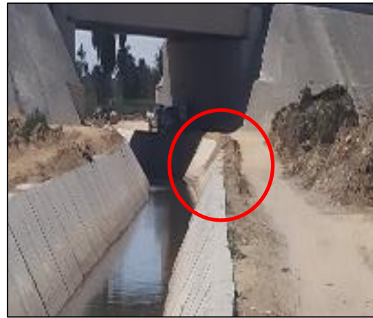
Photo (5): Sliding in some lined slabs
