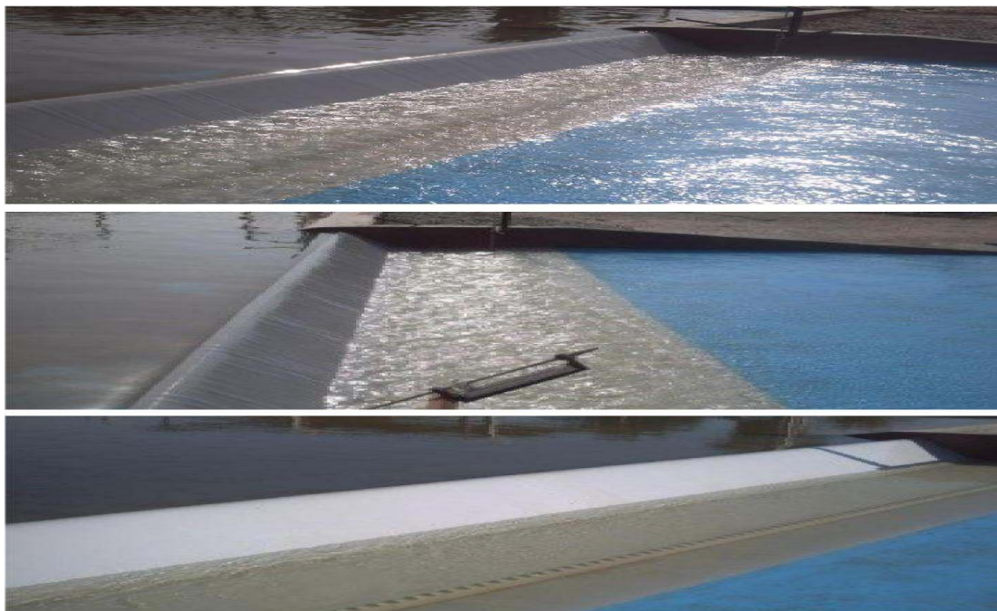
Figure 19. The hydraulic jump within the stilling basin with different discharges.
