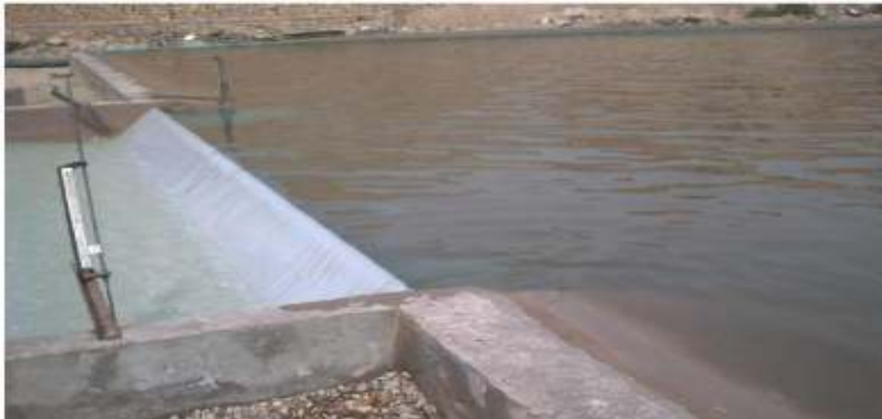
Figure 10. Approach flow to the spillway.
