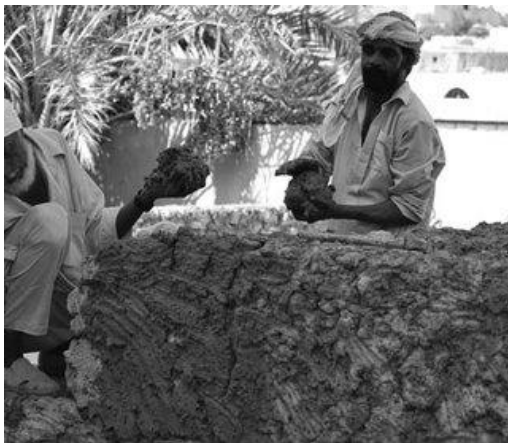
Fig. 7 Vernacular builders in Siwa Oasis using (kershef) and mud.
