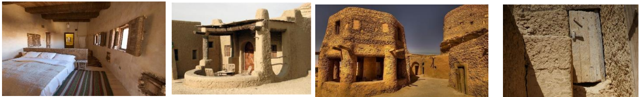
Fig. 5 Using Olive wood and palm trees for making doors and windows
