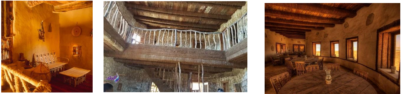
Fig. 4 Using Olive tree trunks were used for the roof.
