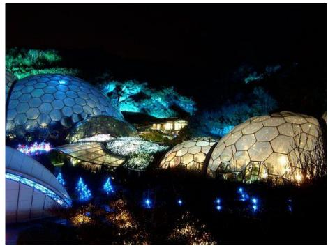
foil) suspended on steel structures to cover 2.2 hectares. The construction of the design was based on the most stable forms on the ground while providing maximum strength with minimum materials. The interior of the domes provides different growing conditions for plants, and the multiple domes of each have a environment different from the other as can also be seen on the screens installed inside, For example, a tropical dome
