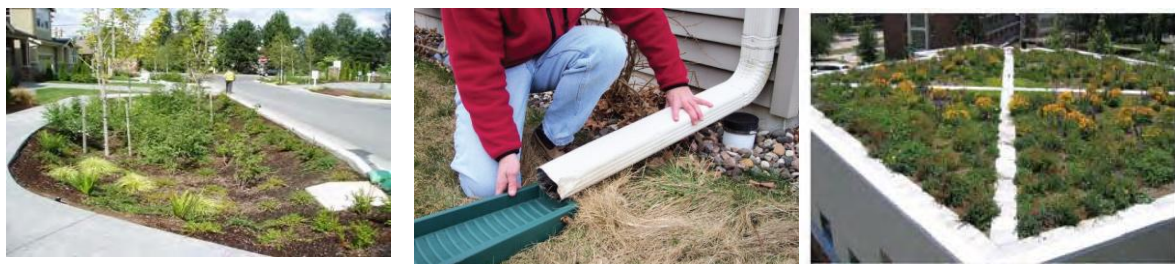
Figure 12 Rain Gardens (Left), Green roofs (Middle), Downspot Disconnections (Right) (Governor's Office of Planning & Research, 2010)
