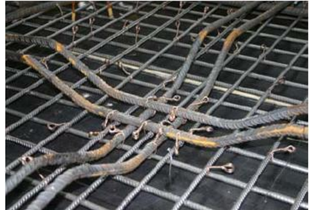
Figure (3) Bent up bars for ductility enhancement.
