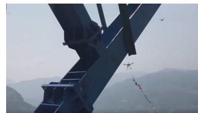
Fig. 5 The drone carrying a cable between the bridge's two towers [23].
