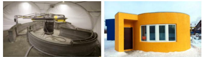
Fig. 14. House during printing process (left) final product after finishing and painting[45].
