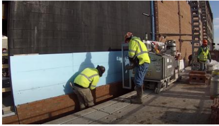
Fig.12. The SAM 100 requires human workers to finish the work [32] .
