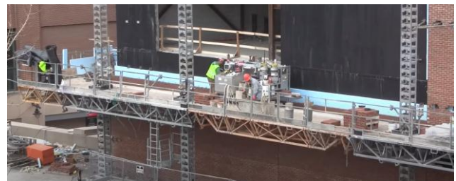
Fig.11. The SAM 100 work on vertical platform[32] .
