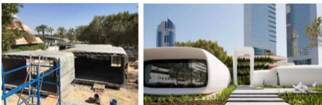
Fig. 13. 3D printed building parts assembly(left) office building after finishing(right)[44].
