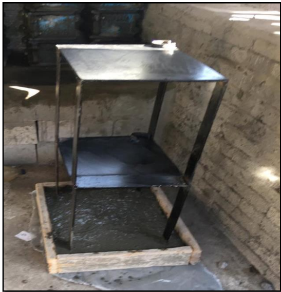
Figure 2 A 2-story space frame (Laboratory Model) during placement of concrete for foundation slab.
