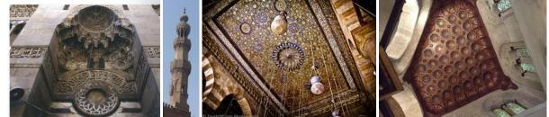
Figure (20): Different structural connection elements in Mamluk religious buildings, left to right: 1-Muqarnas in the portal of Ahmad al-Mihmandar Mosque, 2- Shoulders in the minaret of Qadi Zayn al Din Yahya Madrasa, 3,4- Wood ceilings: (Qibla Iwan in complex of Sultan al-Ghuri, the Mausoleum in Madrasa of Sultan Qala'un. [Author]
