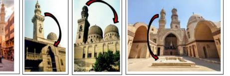
Figure (15) Types of connections between the Minaret and building components, left to right: 1- Complex of Sultan al-Ghuri (Minaret-Street), 2- Minaret of Sultan Barquq Madrasa and Minaret of Sultan Qalaun complex, 3- Mosque of Taghribardi (Minaret-Entrance), 4- The khanqah of Amir Sanjar al-Jawli. (Minaret-Dome), 5- The courtyard of sultan al Nasir Mohamded and Minaret of Sulta Qalaun. [(1) [Behrens-Abouseif, 2007], (2,3,4,5) [Author]].
