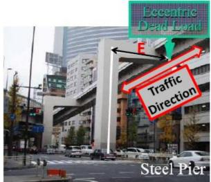
Figure 2: Steel C-Bent Bridge Pier
