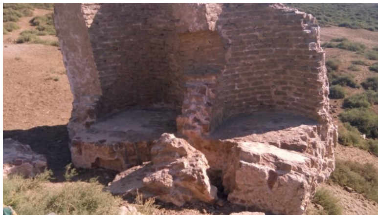
Figure (14): The remains of a building at the south-east side of the dromos (Authors' photograph).
