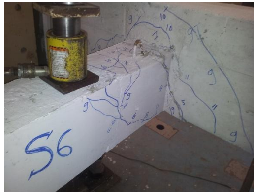
Fig. 15: Specimen-S6 crack pattern at failure
