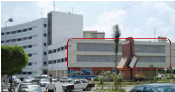
Fig.25 Incorrect architecture shade treatment in north Elevation
