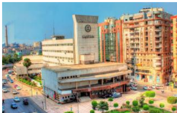
Fig.27: Existing condition for case study Building
