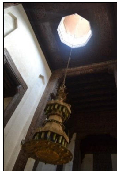
Figure 16 Section in the Shokhshekha used as a natural ventilation inducer in the case study house.
