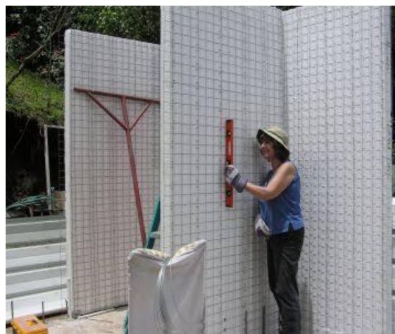
Fig. 2. M2-panel wall under construction
