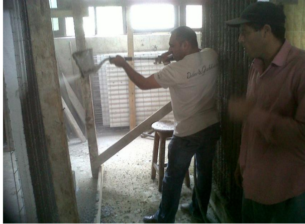
Fig. 5. Application of shot-crete on wall W2
