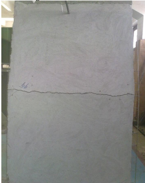
Fig. 7. Failure of Wall W1
