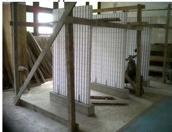
Fig. 4. The three walls before concrete casting
