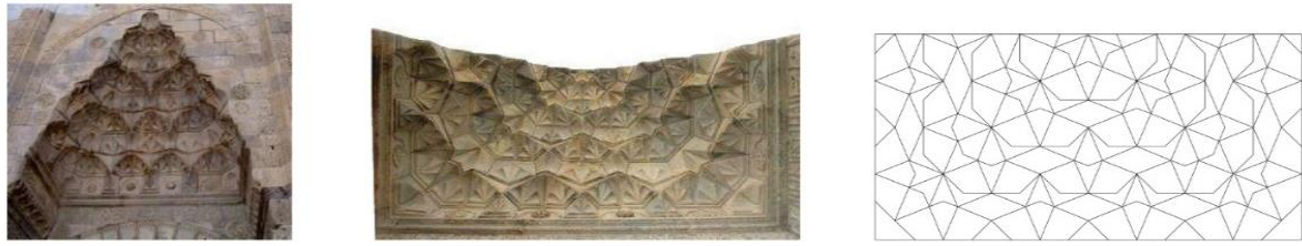
Figure 21. On the left: a view from the front. In the middle: A view from underneath. On the right: plane projections of muqarnas. [11]
