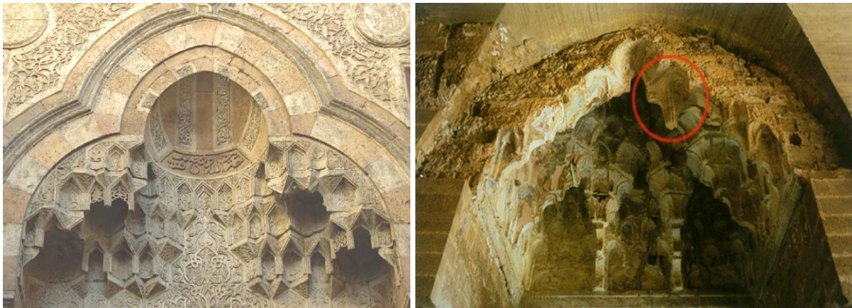
Figure 25. On the left: Muqarnas above the main entrance of the Al-Azhar Mosque in Cairo, Egypt. [42] On the right: Stone muqarnas with hanging elements at the Zisa, Palermo. [43]
