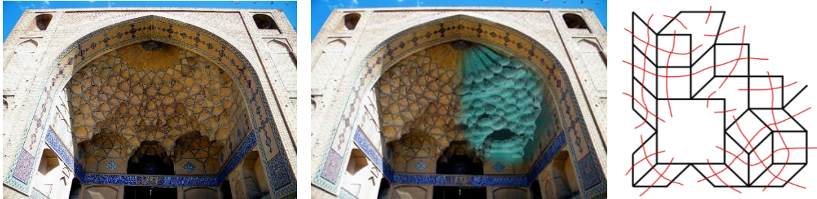
Figure 34. On the left: the portal of the Jame mosque in Isfahan, Iran. [16] In the middle: The colored lines represent the orbits in the muqarnas graph. On the right: Overlay of virtual model and muqarnas.
