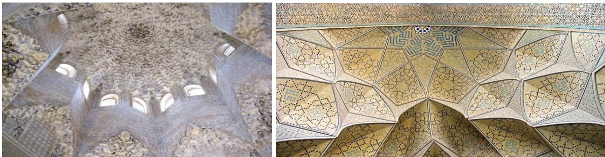
Figure 8. On the left: muqarnas elements in the Imam al-Dur Dome.[23] On the right: the muqarnas decoration on Qazveh Jame mosque in Central Asia. Muqarnas is made with small square tiles, mosaics, calligraphy, which are integrated into the muqarnas.[24]
