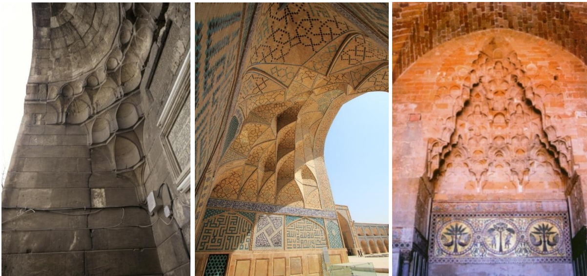
Figure 10. On the left: A transition layer from a dome to a right-angle corner. In the middle: Masjed Jame, Isfahan, Iran. On the right: The muqarnas of the central niche of the iwan in the Zisa, Palermo. [5]
