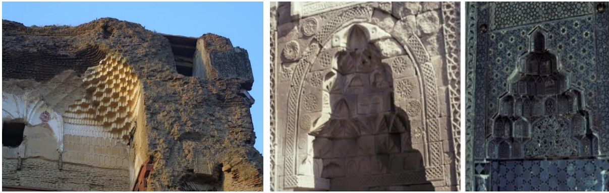
Figure 27. On the left: Old muqarnas through the stone.[46] In the middle: corbeled muqarnas. On the right: superimposed muqarnas.
