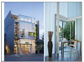
Fig. 10: Example of the application of aerogel in polycarbonate sheets in a multifunctional building in Seattle, Washington's Freemont District<sup>(1)</sup>.
