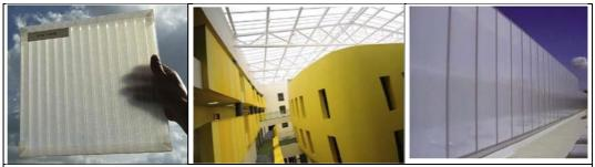
Figure 13: Application of aerogel-filled glazing panel on roof and walls of office building. (a) Aerogel-filled polycarbonate glazing unit; (b) Application on roof; (c) Application on wall <sup>(10)</sup>.
