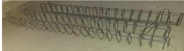
Fig.2: Reinforcement for beams
