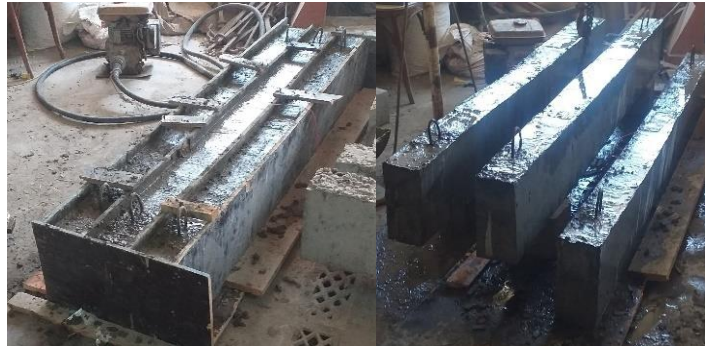
Fig. 3: Casting and curing
