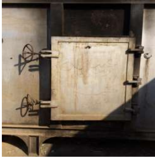
Figure 2: Incinerator main door
