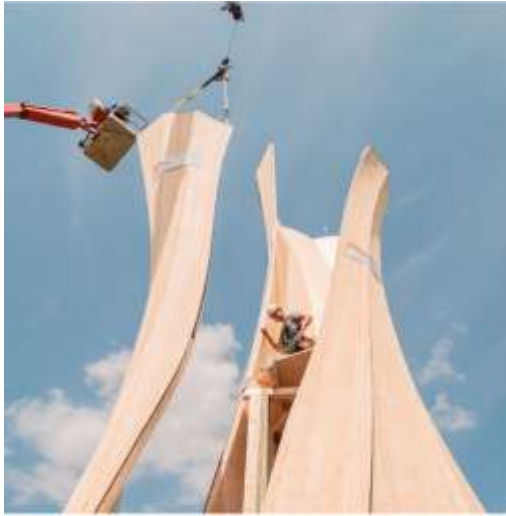
Figure 2: Urbach tower panels during installation (Urbach et al., 2020).
