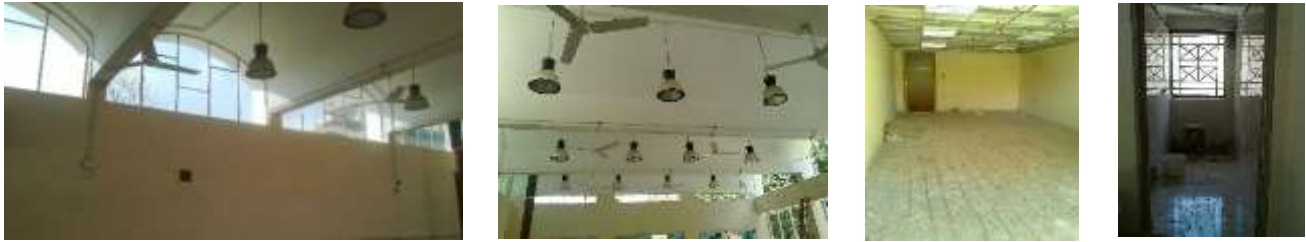
Figure 15: shows the interior biofuel building finish materials during renovation work
