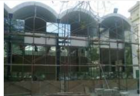
Figure 13: The Double glazed Curtain wall main north façade during renovation
