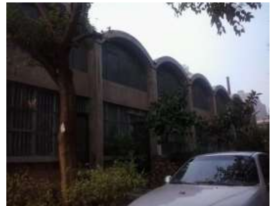
Figure 9: The metal workshop before renovation
