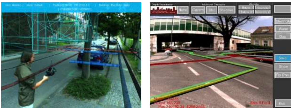
Fig 5. Using Vidente System in generating the 3D underground infrastructure networks via handheld AR device at average depth from 3.0 to 4.0 m.
