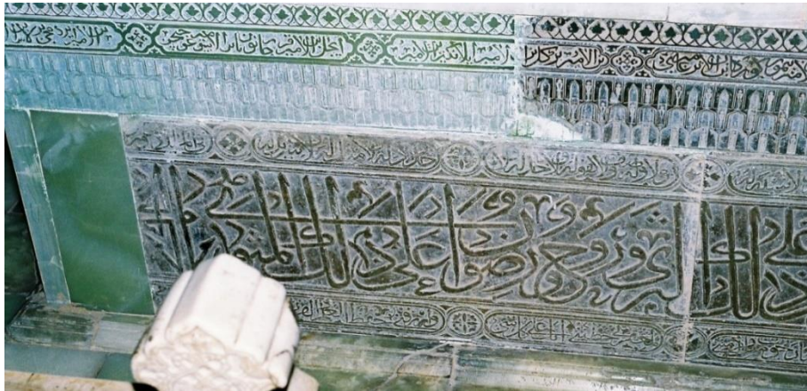
( Plate 6a )Writings on the long northern side of the structure of Amir Zada Mohamed Sultan
