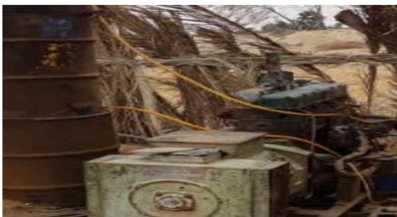
Fig. 1. Diesel energy water pumping system
